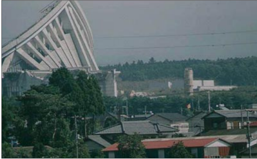
All five columns at the entrance of the Grand Main Temple have been toppled.
