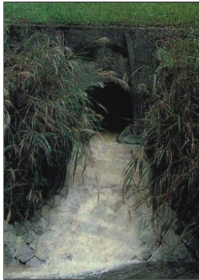
A detail of the circled section at right shows brown waste water from the demolition site flowing into the Urui River.
